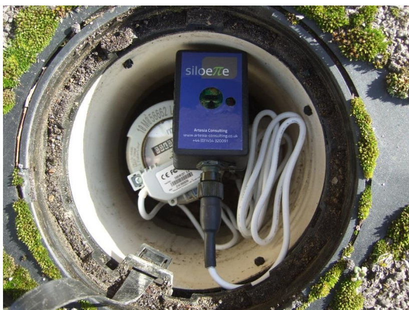
Figure 4 Siloette logger installed in a boundary box
