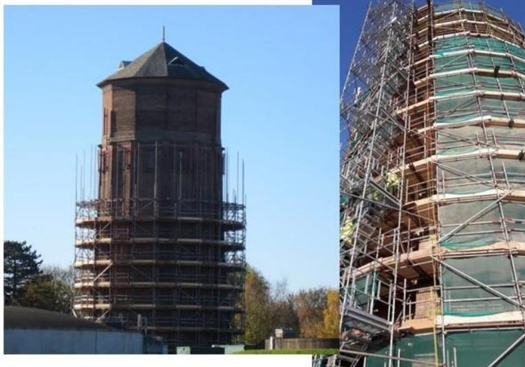
The first part of the project involved erecting scaffolding around the tower, after which the brickwork and roof tiles were inspected to assess the full extent of the repairs required. We also repointed 700m<sup>2</sup> of the brickwork on the south and west sides of the tower, which have more exposure to the prevailing winds. We completed the work on the tower in March this year.
