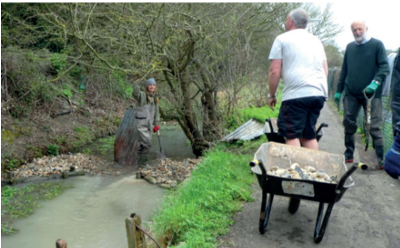
Installing flow deflectors
