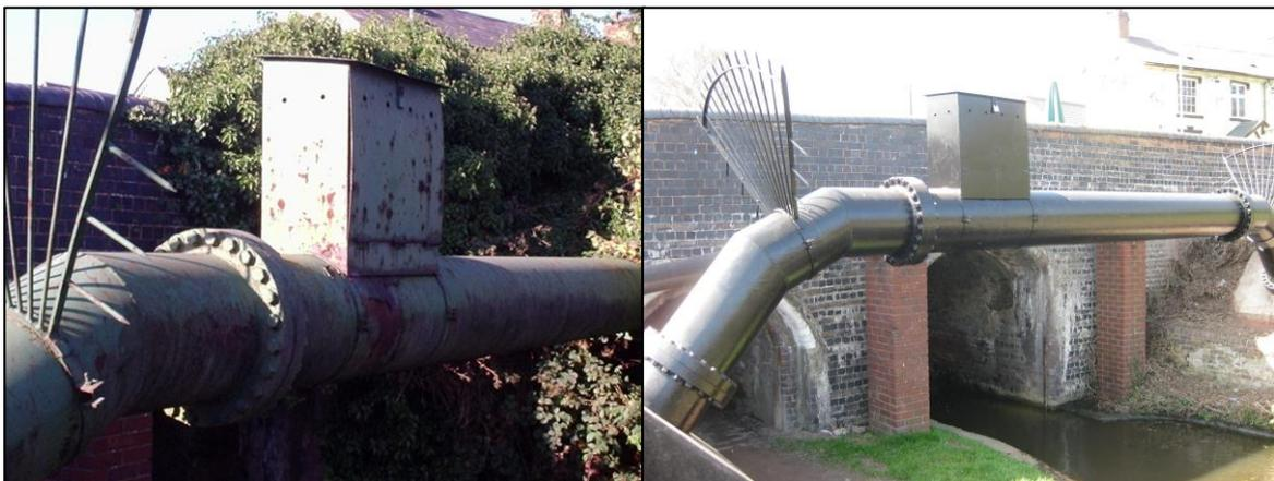
*Figure 6: Kinver lock pipe bridge before and after refurbishment (included replacement riser/air valve, new cabinet, complete blasting and recoat with epoxy)*
