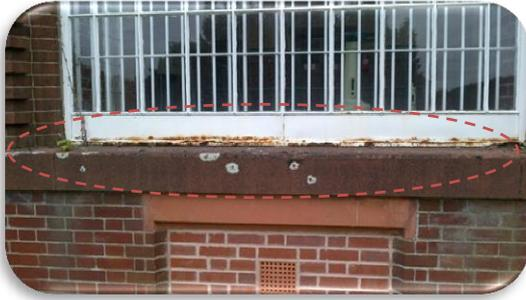
The example shown above in picture W2 has been assessed as in 'poor' condition, this is due to the level of rust present throughout. The window cannot be repaired as with example **W1** and has been identified to become structurally unsound during AMP6. The windows highlighted in this example were installed in 1933 and have exceeded their life expectancy.
