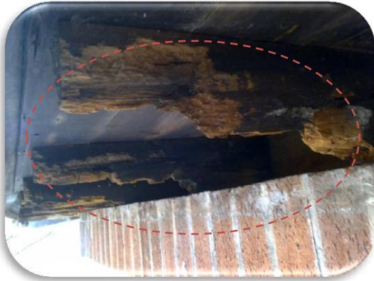
Example **R3** shows a requirement for important remedial interventions in AMP6. The structural beams to this roof are rotten and without interventions in AMP6 it is forecasted that the structure of this roof will fail, producing unacceptable risks to operational assets and the safety of employees.
