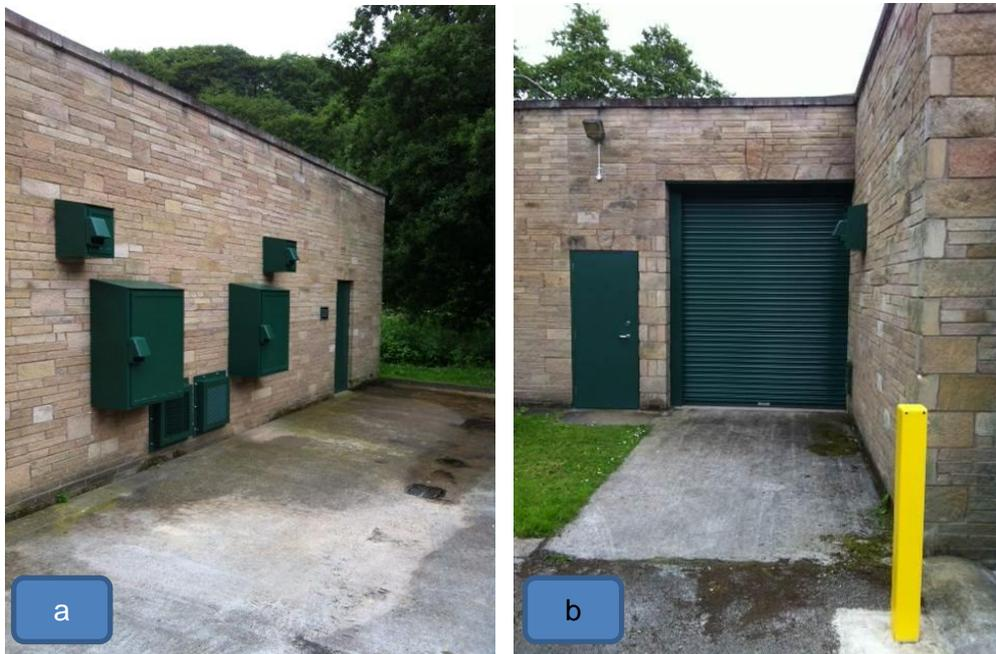
The security solutions detailed above have been installed to protect access points (a - doors and shutters) and to protect chemical delivery points and vents. Electronic solution (b - building alarms and CCTV have also been installed to provide early detection of access to a site and verification at an alarm monitoring centre to instigate appropriate operational and/or Police response.
