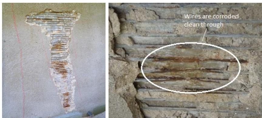
To restore the asset to service will require installation of new post tensioning wires along with new overlay material at an estimated cost of £305k.
