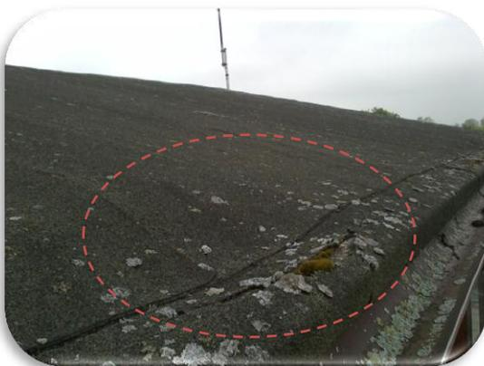
The roof lining on this building has deteriorated significantly during AMP5 and is causing incorrect rain water run-off. Interior leaks have been identified, damaging the interior walls. This roof has been acknowledged for investment in AMP6 in order to negate total roof failure. Preventative repairs have been made and its condition is being managed until refurbishment in AMP6.
