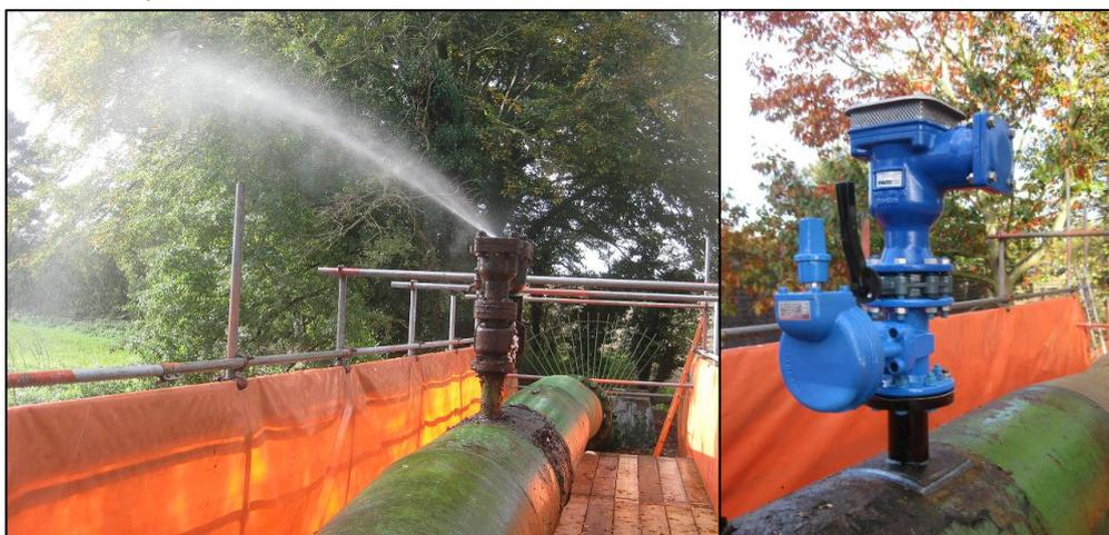
Figure 5: example air valve – pre and post intervention
