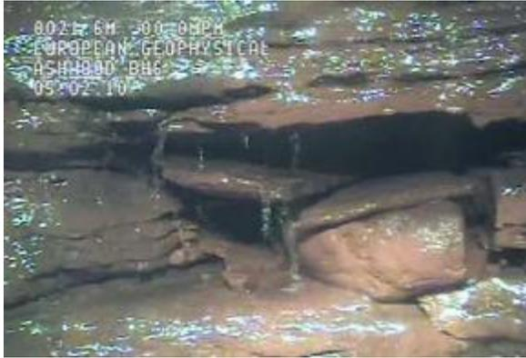
CCTV surveys in February 2010 have shown the existing boreholes to be in poor condition with fissures present at various depths.
