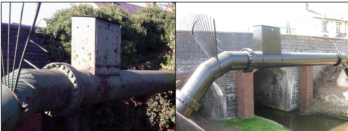
*Figure 6: Kinver lock pipe bridge before and after refurbishment (included replacement riser/air valve, new cabinet, complete blasting and recoat with epoxy)*
