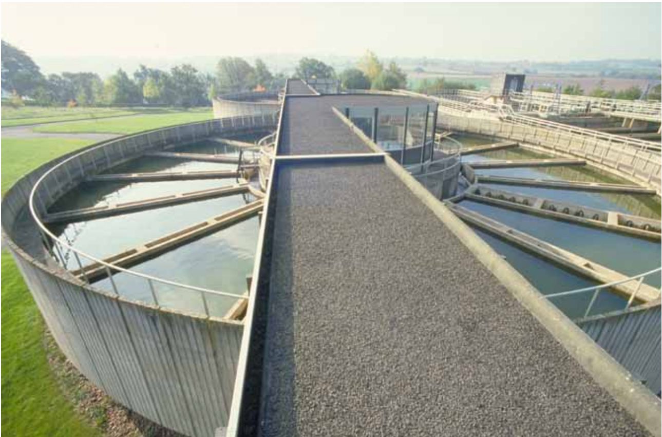
Water treatment at Hampton Loade
