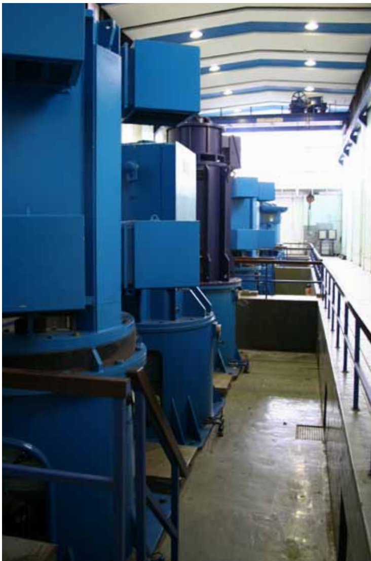
Pumps at Hampton Loade
